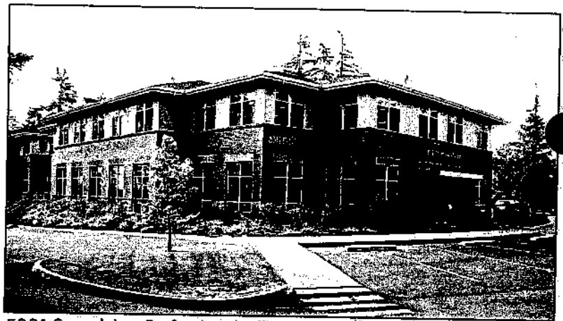
5801 Soundview Professional Office Building
