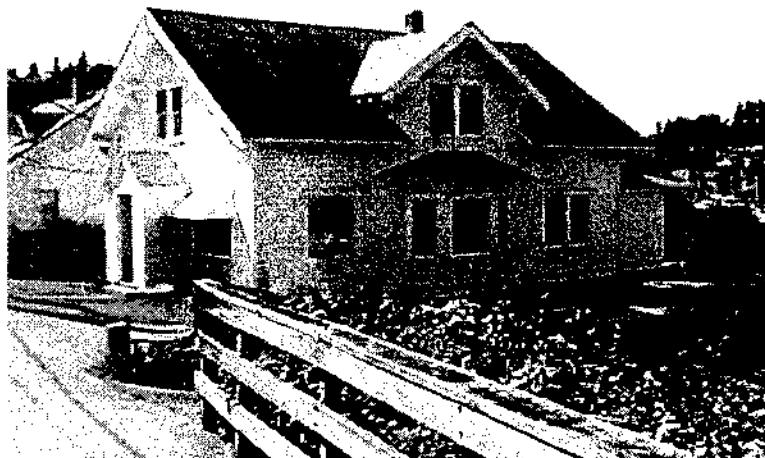
The dominating end-gable and intersecting dormer on the side typify many historic homes in the Gig Harbor basin.
