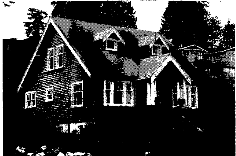
The intersecting dormers and porch gable provide visual interest to this otherwise unbroken roof plane.
