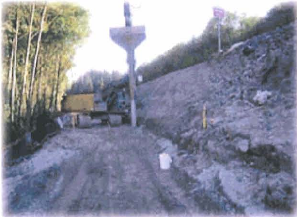
Installation of D-RAP foundation in tight spaces for Phase 2 construction
