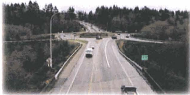
Existing Condition - Photo from Bucket Truck
