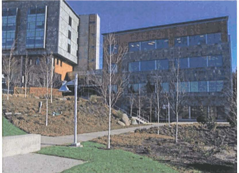
St. Anthony's Regional Hospital, opened 2009, required roadway and interchange improvements as transportation mitigation
