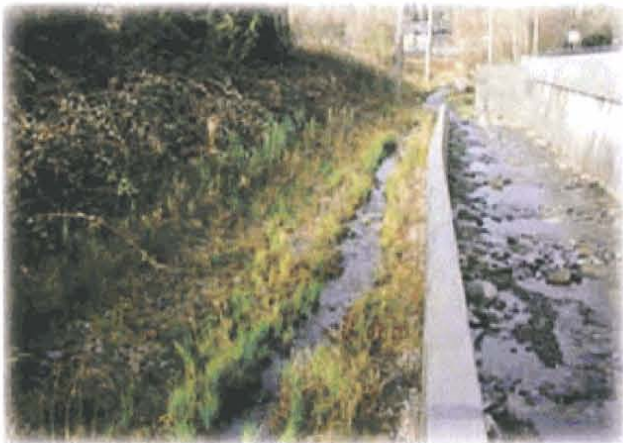
McCormick Creek natural-lined fishway with "rock riffles" addresses a perched culvert condition
