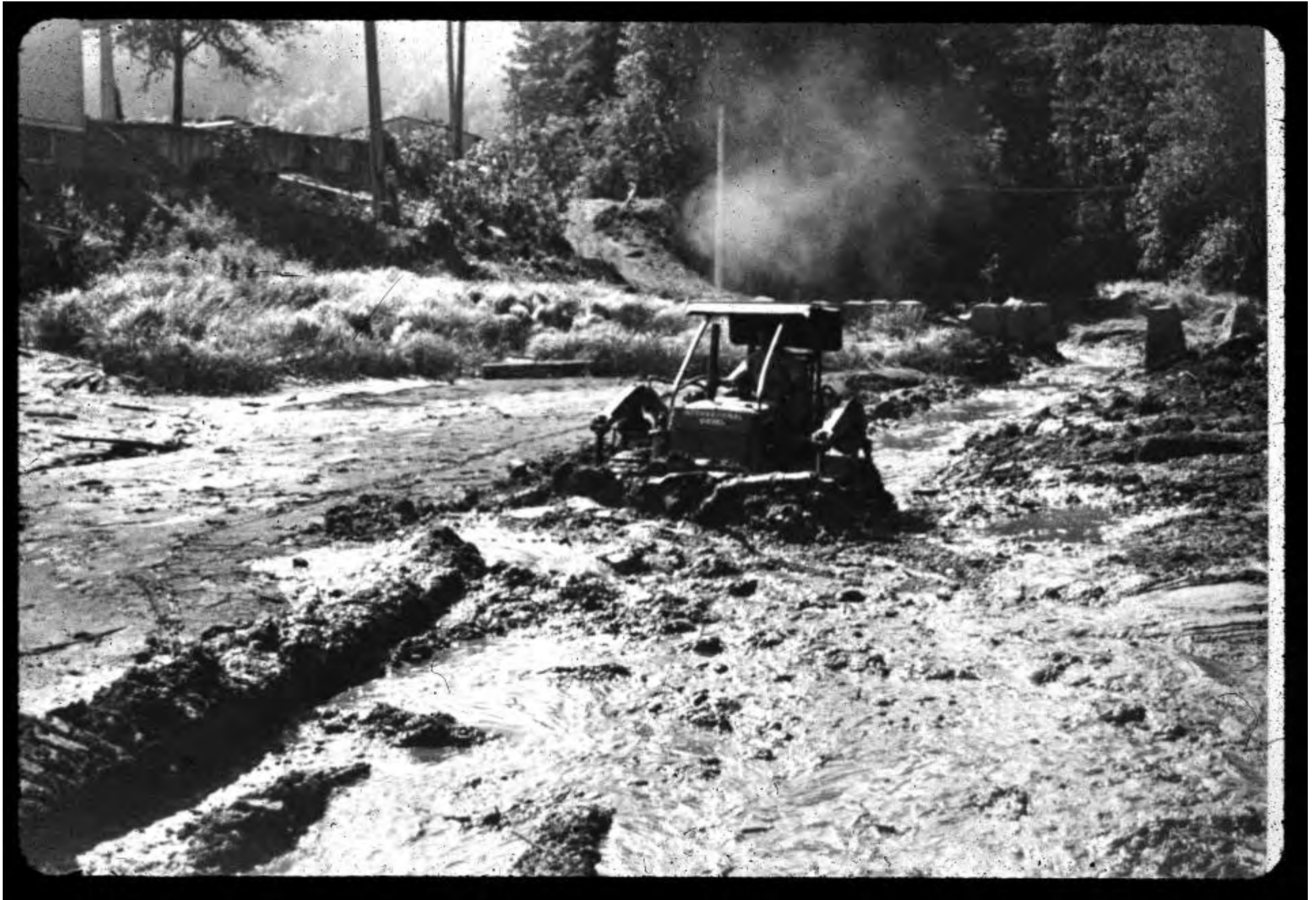
Donkey Creek Mudflats during Pipe Installation
