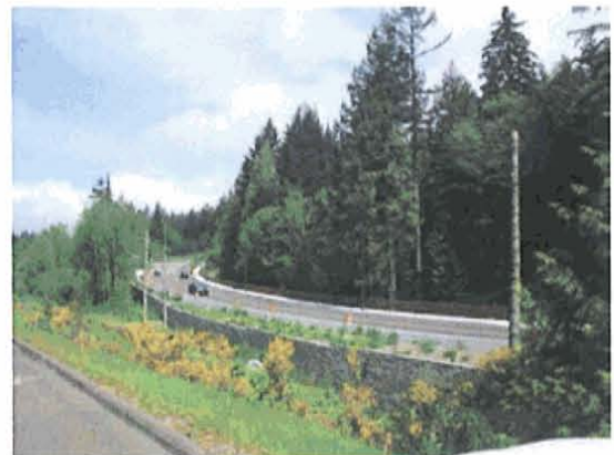
Completed Canterwood Blvd. NW Phase 1 Construction
