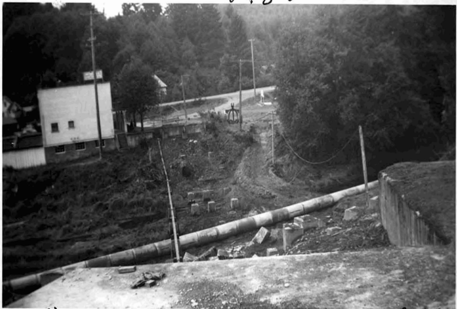
new fill under construction at peninsula light Co
