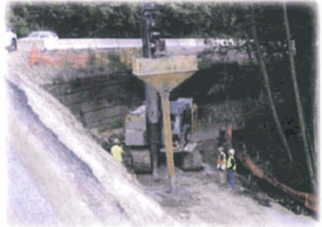
Installation of D-RAP foundation in tight spaces for Phase 2 construction
