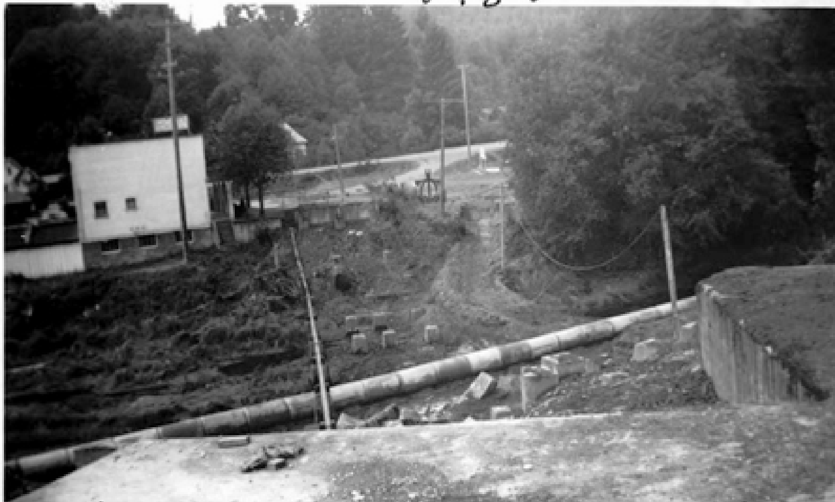
new fill under construction at Peninsula Light Co
