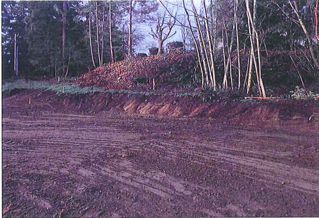
LOT 7/8 FACING SOUTHWEST 02/11/16
