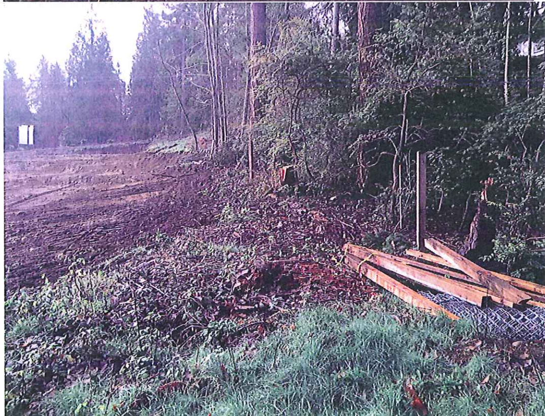
LOT 6/7/8 FACING SOUTH 02/11/16
